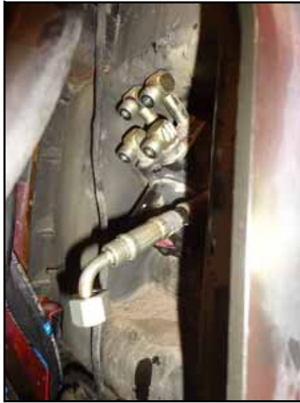
FIGURE 13. Hoses Disconnected from Steering Orbital
