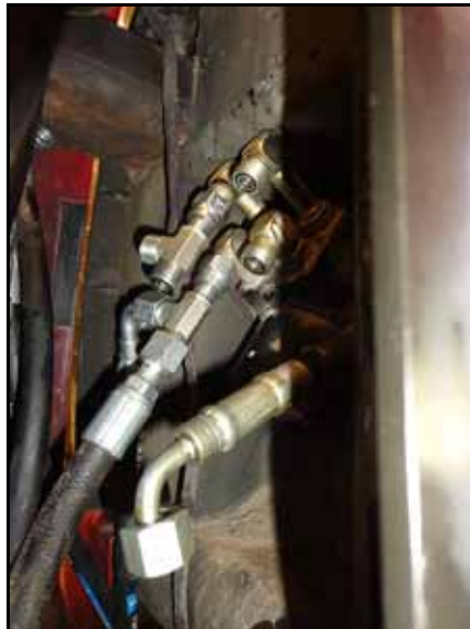
FIGURE 18. Tee Fitting Installed in Tank Port
