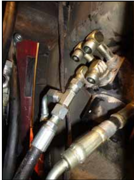
FIGURE 16. Hydraulic Hose Installed on Tee Fitting
