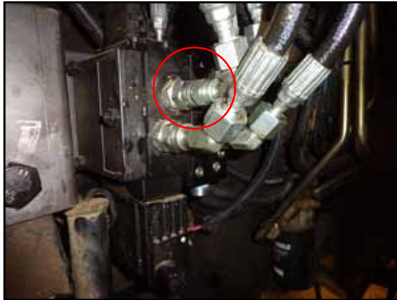
FIGURE 29. Right Hose Installed on Steering Valve
