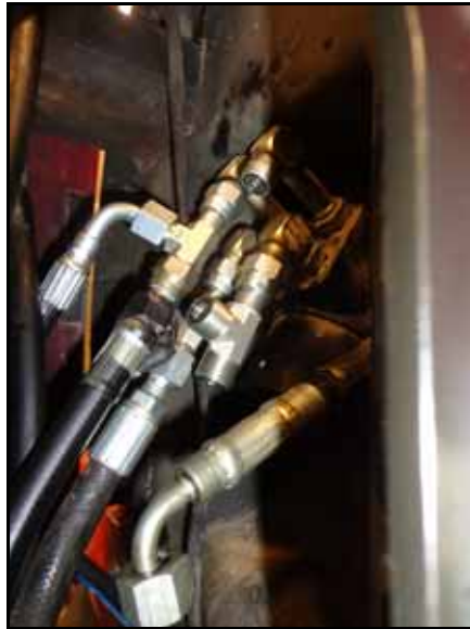
FIGURE 22. Tee Fitting Installed in Right Steering Port
