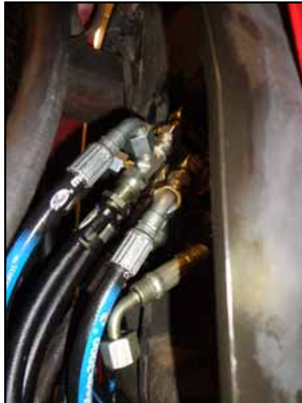
FIGURE 28. Hydraulic Hose Installed on Tee Fitting
