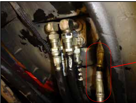
FIGURE 6. Machine's Load Sense Hose
