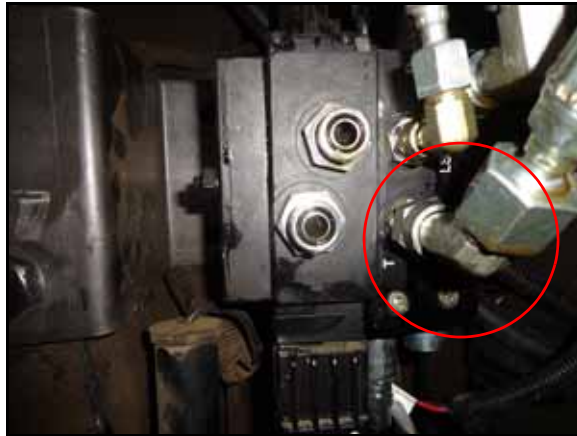
FIGURE 21. Tank Hose Installed on Steering Valve
