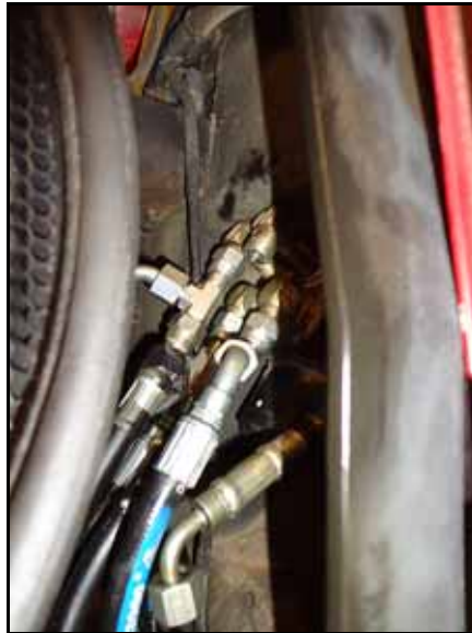
FIGURE 24. Hydraulic Hose Installed on Tee Fitting
