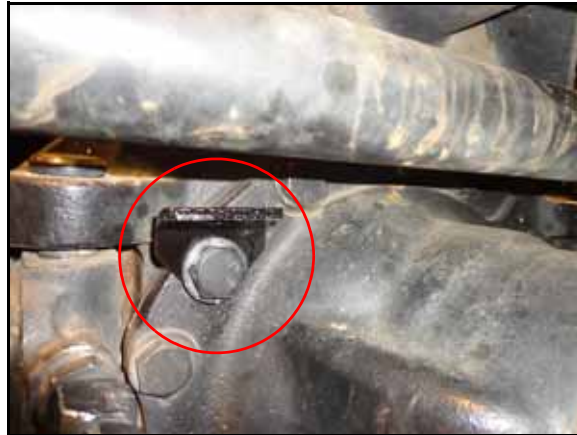
FIGURE 3. WAS Base Mounting Bracket Installed
