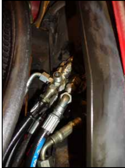
FIGURE 27. Machine's Left Steering Hose Installed
