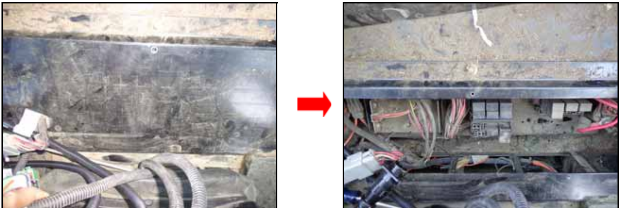
FIGURE 1. Wall Access Plate Removed
