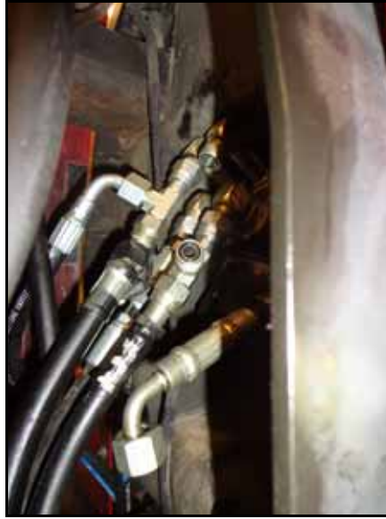
FIGURE 23. Machine's Right Steering Hose Installed
