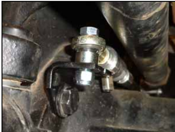
FIGURE 6. Base-End of Sensor Installed on Machine
