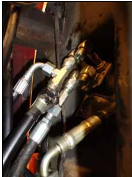
FIGURE 20. Hydraulic Hose Installed on Tee Fitting
